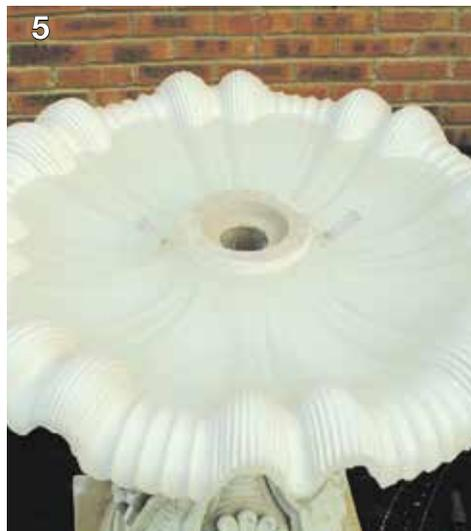
The shell is then levelled and secured with resin. To level the bowl temporarily block the pipe outlets in the bowl, fill with water and level by eye. Do not use a spirit level for this operation. Packers can be used to assist in levelling the bowl. Once the resin has hardened the packers should be removed.
