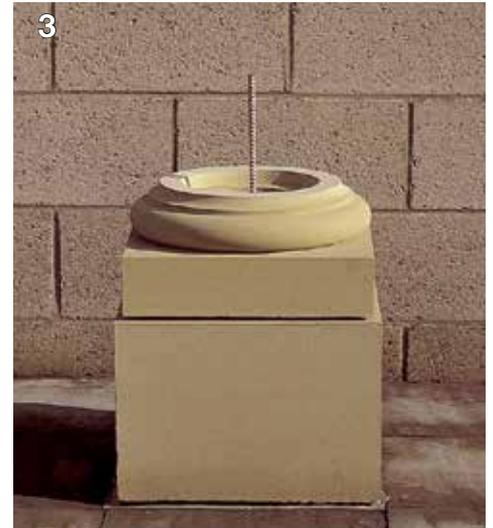
The column base is bedded on the pedestal as previously described.
