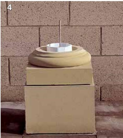
It is important that polystyrene/Styrofoam (or similar) is used to act as an isolating medium between the stone and infill concrete. This is inserted into the core of the pedestal and base. Care should be taken to ensure sufficient overlap at both vertical and horizontal joints with continuous contact between the isolating material and the inner stonework core.
