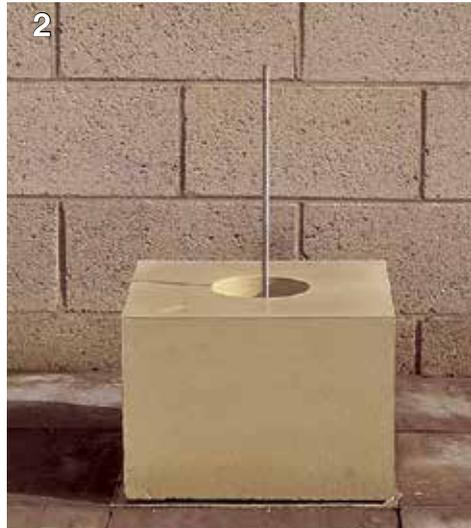
The pedestal is then bedded on 1:1:6 cement/lime/sand mortar. All joints would normally be 6mm (1/4") with the mortar slightly recessed from the surface of the stonework to allow for pointing after the column is erected.
