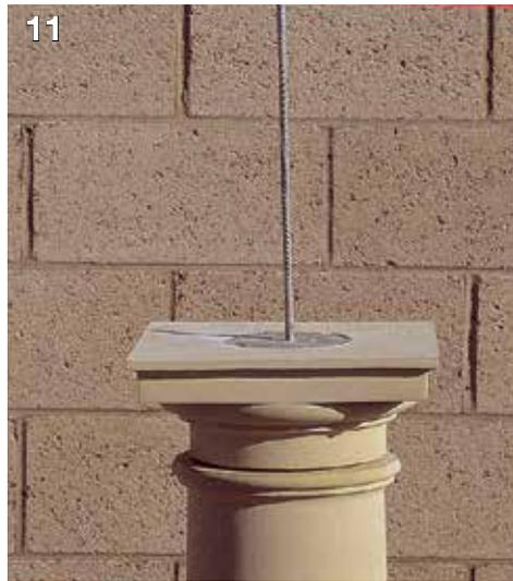
11 Column ~ Entablature or Structure above: the joint around the structural core between the capital and the entablature or structure above should be formed using a compressible filler, or a weak mortar mix, to form a 6mm (1/4") soft joint. This ensures that any loading is carried by the central structural core and not by the stonework.
