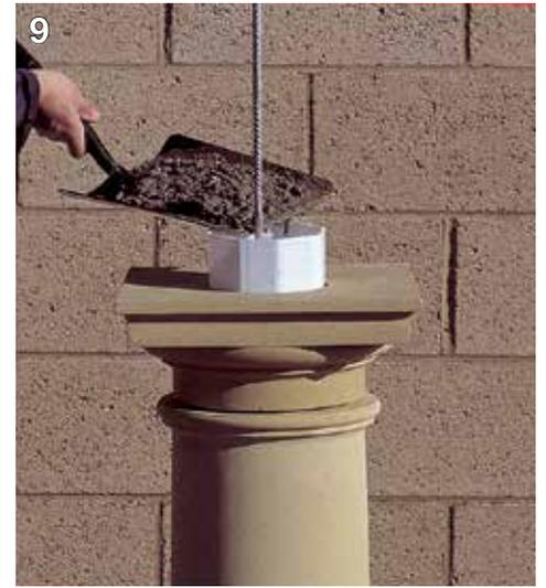
9 The capital is then bedded. The isolating medium is inserted into the core. The core is then partly infilled with concrete as previously described
