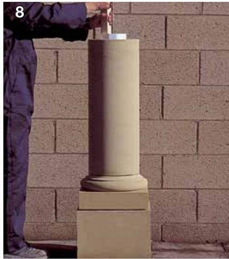
8 The concrete is then hand compacted. The second and third shaft sections being installed in the same way (unless a single shaft unit).
