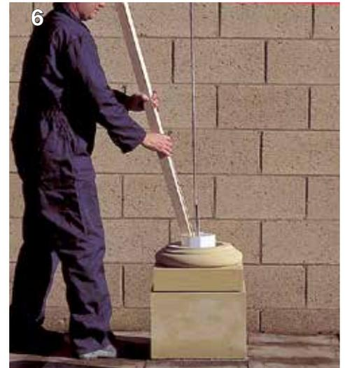
The steel main bar reinforcement is tied to the starter bar insuring sufficient overlap. The concrete is then carefully compacted by hand.
