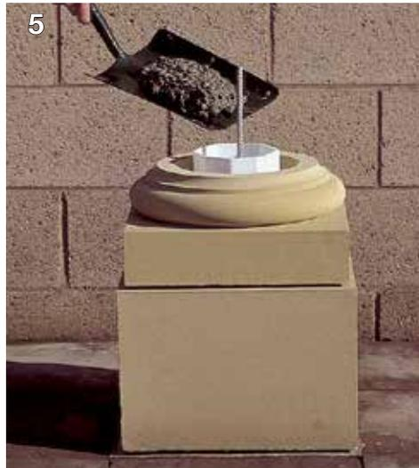
The pedestal and base are then infilled with concrete. The coarse aggregate of the concrete being rounded gravel of maximum 10mm (3/8"). All subsequent concrete pours should only take place after the concrete in the preceding section has reached its initial set.
