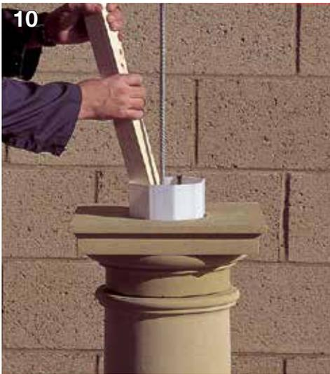
10 The isolating medium is then trimmed flush. Continue concrete infill until level with top of capital. The capital is now ready for the next stage, either (11) or (12).
