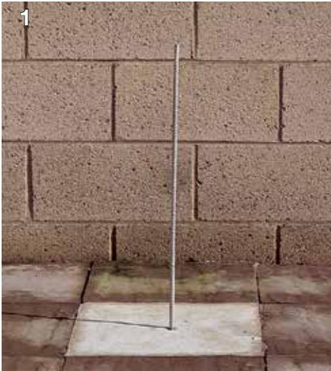
The column should be erected on a suitable foundation. Foundation, concrete and steel reinforcement to be designed by others to suit loadings and ground conditions. Shown is a suitable steel starter bar set into a concrete foundation.
