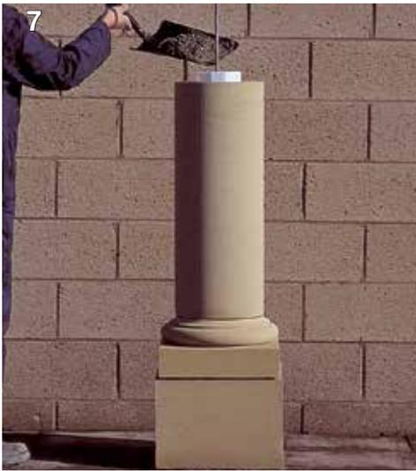
7 The bottom shaft section is then bedded and the isolating medium inserted as previously described. The concrete is again infilled.
