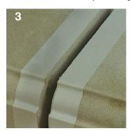
The joint is now ready to start pointing. Please note, with TecStone and TecLite materials, the masking of joints is not always necessary.
