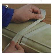
Apply masking tape to both sides of the joint, keeping the tape approximately 1mm (1/16") from the edge of the joint.
