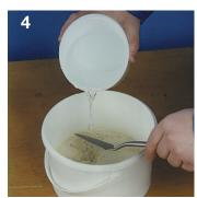
Carefully add small quantities of water to the Haddonstone pointing mix, mixing thoroughly to ensure the water is fully dispersed. \*See note below.
