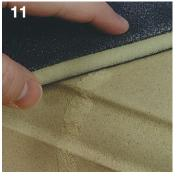
Any mix residue may be rubbed The finished joint. away with fine abrasive paper 2-3 days after completion.
