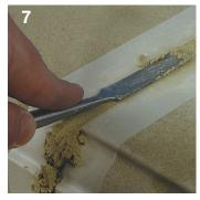
Smooth the pointing mix to the profile of the stone, removing any excess pointing mix.
