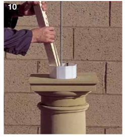
The isolating medium is then trimmed flush. Column ~ Entablature or Structure above: the Column ~ Freestanding or timber pergola: the Continue concrete infill until level with top of joint around the structural core between the capital. The capital is now ready for the next capital and the entablature or structure above stage, either (11) or (12).
