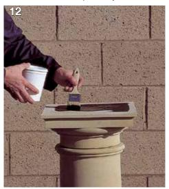
top of the capital will need to be waterproofed, as a minimum, with bituminous paint (applied in accordance with manufacturers instructions) to approximately 25mm (1") from the edge of the
