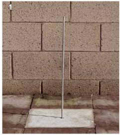
The column should be erected on a suitable The pedestal is then bedded on 1:1:6 cement/ The column base is bedded on the pedestal as reinforcement to be designed by others to suit 6mm (1/4") with the mortar slightly recessed from loadings and ground conditions. Shown is a the surface of the stonework to allow for pointing suitable steel starter bar set into a concrete after the column is erected. foundation
