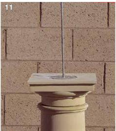
should be formed using a compressible filler, or a weak mortar mix, to form a 6mm (1/4") soft joint. This ensures that any loading is carried by the central structural core and not by the stonework.
