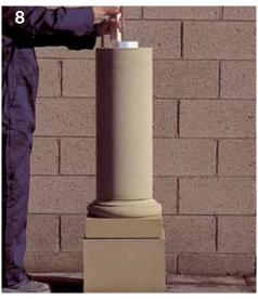
The concrete is then hand compacted. second and third shaft sections being installed in the same way (unless a single shaft unit).
