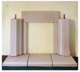
Mark out the required position of the fireplace legs and the optional slips to suit your fireplace and fire opening. Attach both legs to wall using 100 x 25mm (4" x 1") mild steel straps as shown and bed on 1:1:6 cement/lime/sand mortar. Install the slip blocks with a proprietary resin mortar at the required spacing.
