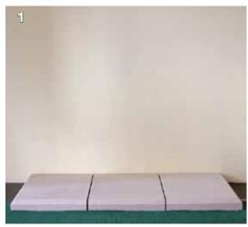
The hearth blocks should be bedded on a suitable base using a 1:1:6 cement/lime/sand mortar. All joints would normally be 6mm (¼") with the mortar slightly recessed from the surface of the stonework to allow for pointing after the fireplace is installed.
