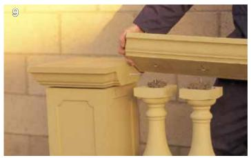
Mark and drill the underside of the rail to create 16mm (%) holes ready for balusters at desired spacing  $\sim$  enlarge holes if necessary to allow for installation tolerance. Also drill and resin 6mm ( $\frac{1}{4}$ ) dowels to both ends of the rail. Final assembly of this section can now take place with the rail being bedded on a mortar bed.
