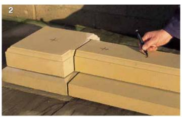
Mark the pier base centrally and drill a 20mm (%") hole through the pier base and pier undercoping and into the foundation. Similarly, the undercoping and plinth should be drilled to a diameter of 10mm (%") and dowelled twice per stone into the foundation. Ensure that holes are positioned so that they will eventually be hidden by balusters.
