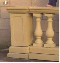
The finished balustrade is then ready for pointing. For details refer to the Pointing Recommendations sheet.
