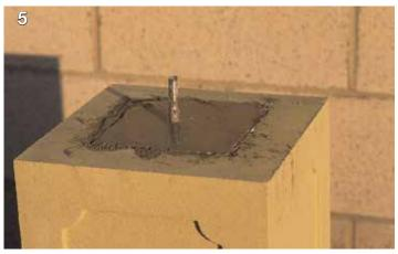
The isolating/expansion material is trimmed and the concrete trowelled so that both are flush with the top of the shaft. Insert 10mm (%") stainless steel dowel 100mm (4") long minimum into top of concrete, to protrude by 40mm (1½"). Only proceed once concrete has reached its initial set.
