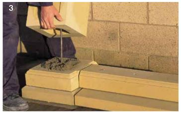
Resin fix a 10mm (%") stainless steel dowel positioned to extend 300mm (12") above the pier base. The pier shaft can then be bedded, using the method previously described.
