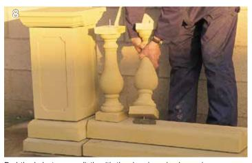
Bed the balusters on plinth with the dowels resined ensuring any seam marks run lengthways along the plinth.
