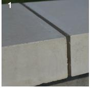
Before pointing ensure each 6mm (1/4") joint is free from loose particles. Avoid pointing in extreme conditions, particularly wet and cold.
