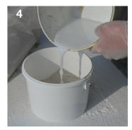
Carefully add small quantities of water to the TecStone pointing mix, mixing thoroughly to ensure the water is fully dispersed. \*See note below.
