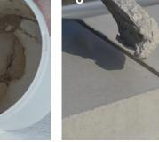
Scoop the mix into the joint, pressing with a trowel to ensure an even fill.
