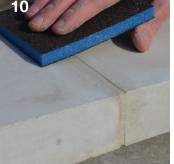
Any mix residue may be rubbed away with fine abrasive paper 2-3 days after completion.
