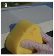
Wipe over the surface of the joint and surrounding area with a dampened sponge to remove all surplus pointing material off the surrounding areas and ensure a flush finish to the joint.
