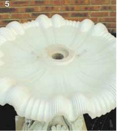
Temporarily support the fountain bowl above The shell is then levelled and secured with resin. the shaft ensuring the design on the bowl lines To level the bowl temporarily block the pipe up with the design on the support. Connect the outlets in the bowl, fill with water and level by plumbing and feed down through the core of the eye. Do not use a spirit level for this operation. Packers can be used to assist in levelling the bowl. Once the resin has hardened the packers should be removed.
