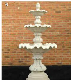
Subsequent levels are installed as previously described, again ensuring the design on the bowl and the supports line up and that the bowls are level. Once the stonework is installed the pump and plumbing should be connected as described on the relevant Tech Sheet. The valves and pump should be set to minimum before the pump is turned on. Adjustments can be then made to suit your specific fountain, pool and location.
