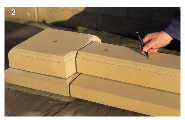
Mark the pier base centrally and drill a 20mm (%1") hole through the pier base and pier undercoping and into the foundation. Similarly, the undercoping and plinth should be drilled to a diameter of 10mm (%1") and dowelled twice per stone into the foundation. Ensure that holes are positioned so that they will eventually be hidden by balusters.
