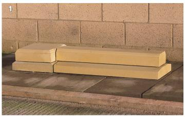
The balustrade should be erected on a suitable foundation. The foundation, concrete and steel reinforcement to be designed by others to suit loading and ground conditions. Shown is a pier base, pier undercoping, plinth and an undercoping bedded on 1:1:6 cement/lime/sand mortar. All joints would normally be 6mm (1/4") with the mortar slightly recessed from the surface of the stonework to allow for pointing after the balustrade is erected.
