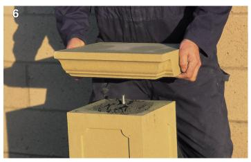
Drill a 20mm (%") hole in underside of pier cap and drill a 16mm (%") hole in the side of the pier cap at the rail run-in ready for the rail installation. Resin dowel and bed the pier cap on a continuous mortar bed on the pier shaft.
