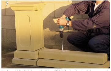
Mark and drill plinth to create 16mm (5%") holes to allow for tolerance ready for balusters at desired spacing in accordance with Tech Sheet B70
