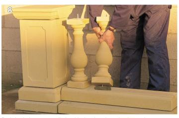
Bed the balusters on plinth with the dowels resined ensuring any seam marks run lengthways along the plinth.
