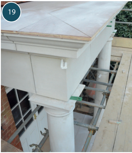
Columns, architrave and cornice all installed. Flat roof in position prior to leading.
