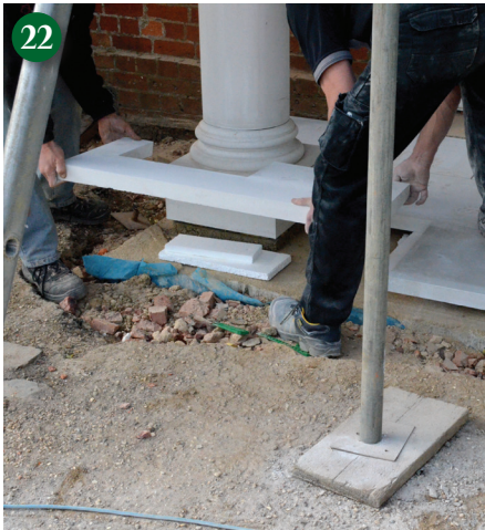
Floor is installed at this point to reduce risk of damage taking place during construction. All cutting done on site.
