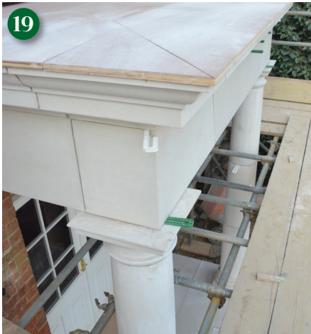
Columns, architrave and cornice all installed. Flat roof in position prior to leading.
