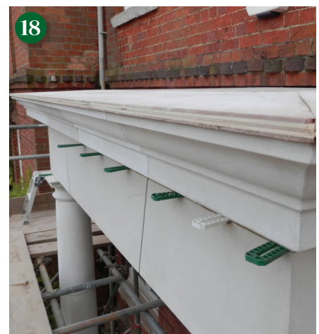
Cornice stones in position with spacers shown.
