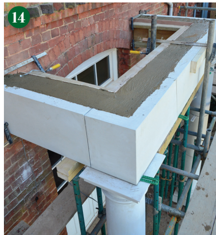
Concrete infill of entablature complete.
