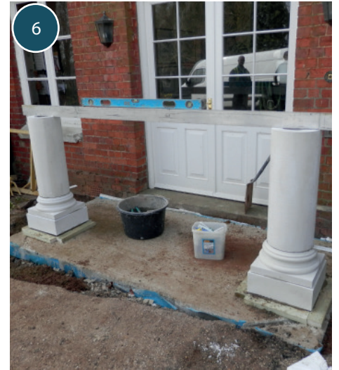
6 It is important to check levels throughout the installation process.
