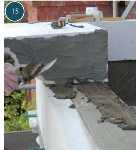
Cornice stone installation underway.
