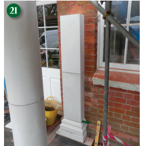
Pilaster shaft sections during installation.
