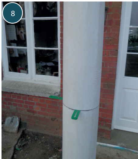
8 Spacers are used to ensure the correct joints, normally 6mm ( \frac{1}{4} ").
