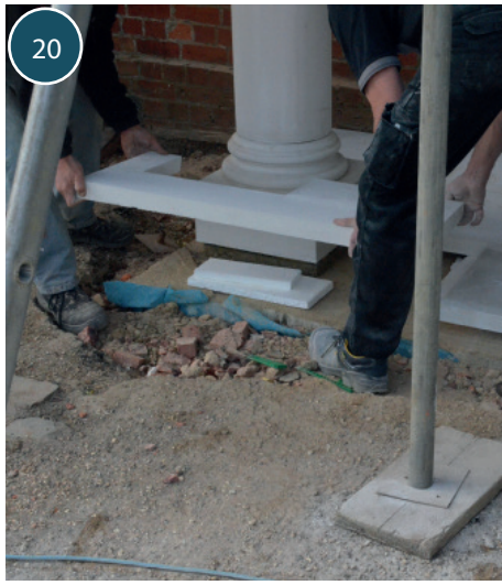
Floor is installed at this point to reduce risk of damage taking place during construction. All cutting done on site.
