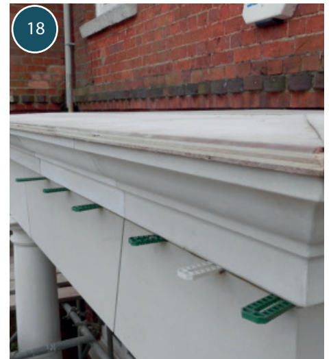
Cornice stones in position with spacers still in position.
