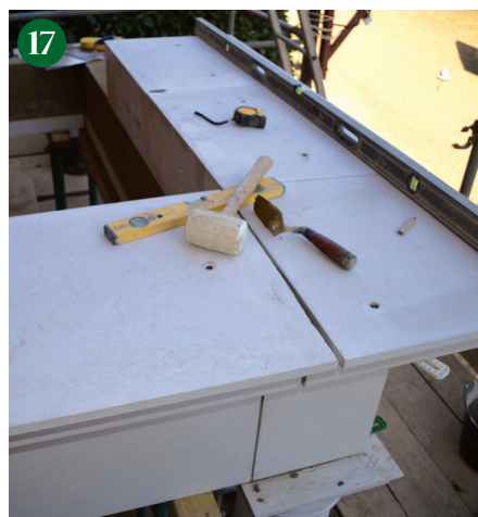
Top view of cornice during installation.
