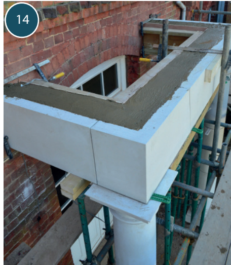
Concrete infill of entablature complete.
