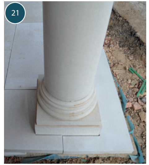
Floor in position prior to pointing.
