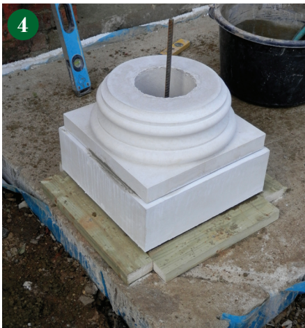
Column pedestal and base bedded on 1:1:6 cement/lime/sand mortar. Starter bar already installed. (Refer to Column Assembly Recommendations for more information).
