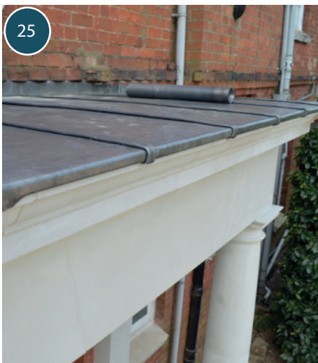
Lead roof installation to ensure waterproof structure.
