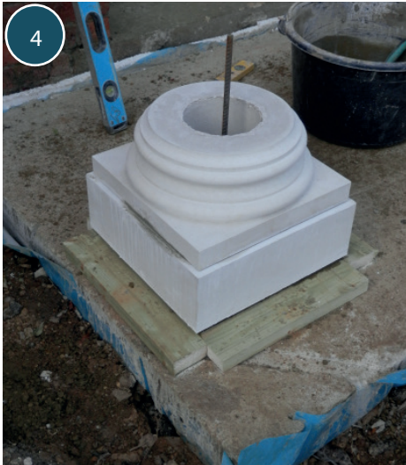
4 Column pedestal and base bedded on 1:1:6 cement/lime/sand mortar. Starter bar already installed. (Refer to Column Assembly Recommendations for more information).
