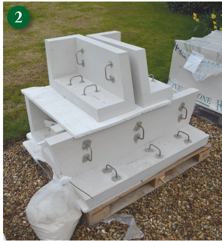
A typical pallet showing architrave stonework featuring 'D' lugs to ease installation.
