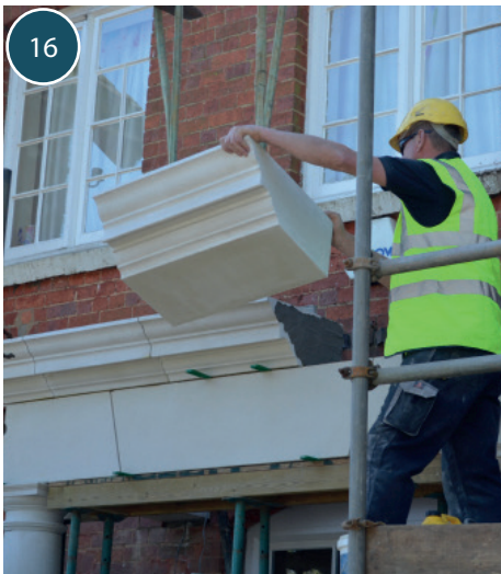
Cornice stones being mechanically lifted into position.
