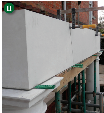
Exterior view of entablature showing supports, spacers and clamps.
