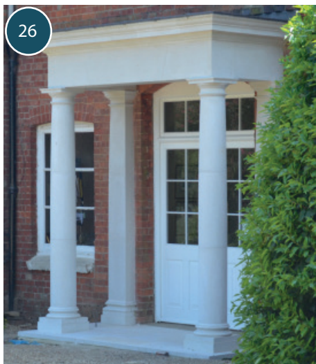
The finished Gibbs Porch with all pointing completed. (Refer to Pointing Recommendations sheet for further details).
