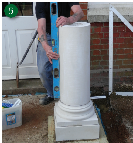
Bottom shaft section bedded on the base as previously described.
