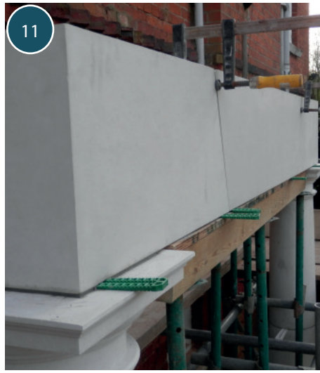
Exterior view of entablature showing supports, spacers and clamps.
