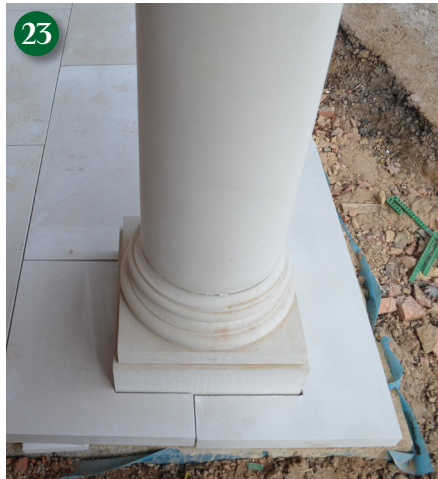
Floor in position prior to pointing.
