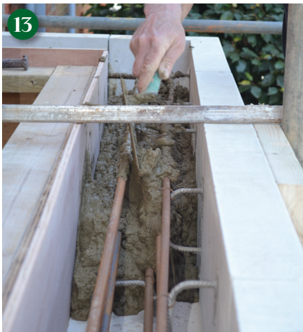
Concrete infill underway.
