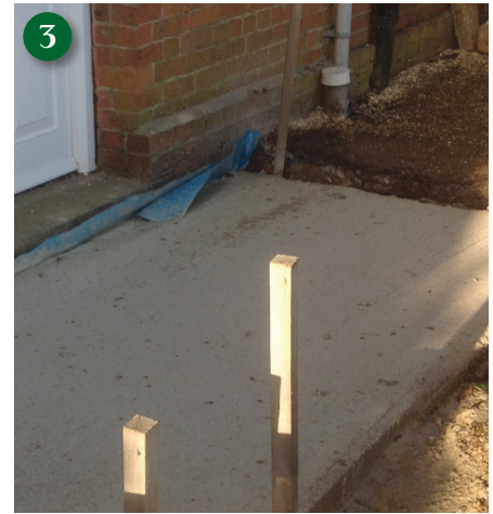
Concrete foundations installed to correct dimensions and specifications (designed by others).
