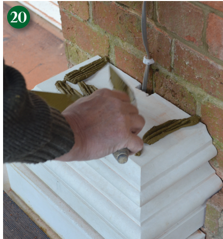
Pilaster base during installation. Note: wiring can be hidden behind these elements if required.
