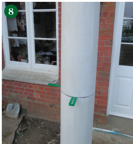
Spacers are used to ensure the correct joints.
