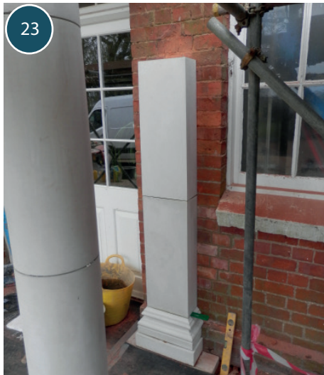
Pilaster shaft sections during installation.
