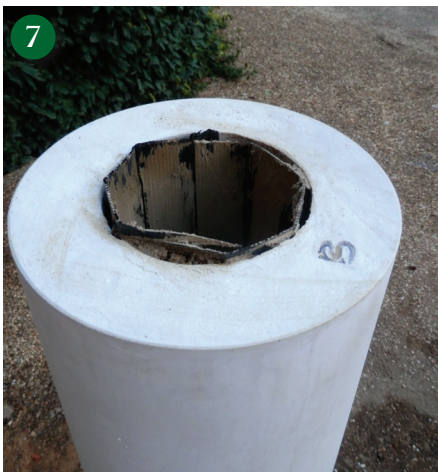
Polystyrene/Styrofoam (or similar) should be used to act as an isolating medium between the stone and infill concrete.
