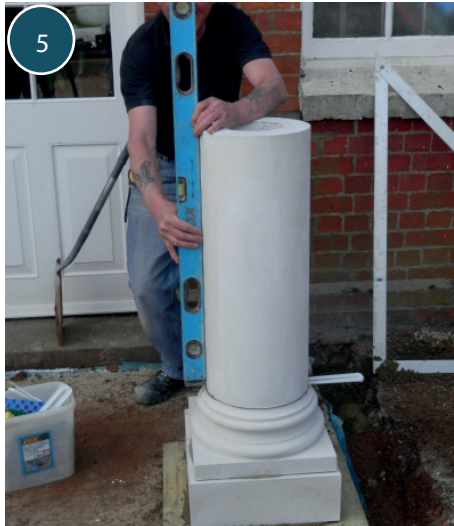
5 Bottom shaft section bedded on the base as previously described.
