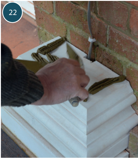
Pilaster base during installation. Note: wiring can be hidden behind these elements if required.
