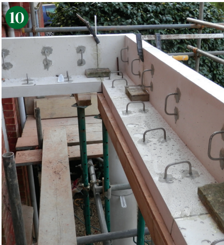
Entablature in position showing 'D' lugs.
