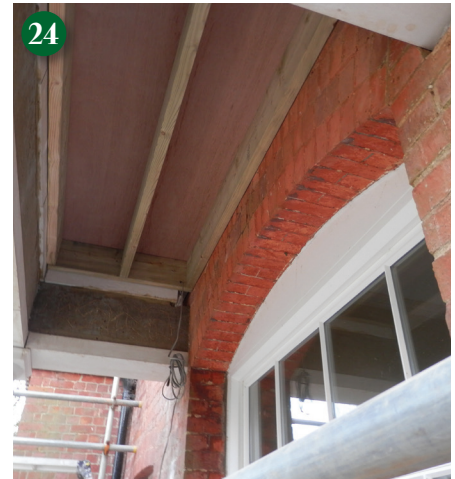
Internal view of roof structure and exposed concrete infill to architrave before finishing.
