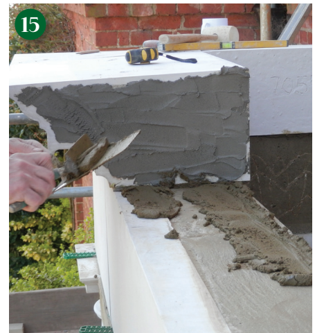
Cornice stone installation underway.
