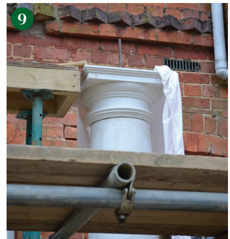
Capital in place with starter bar protruding. Scaffolding must be used when working at higher levels.
