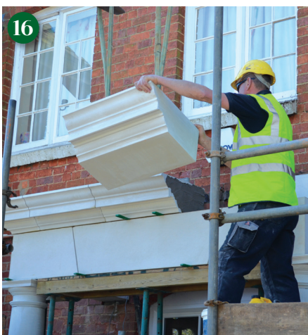
Cornice stones being mechanically lifted into position.
