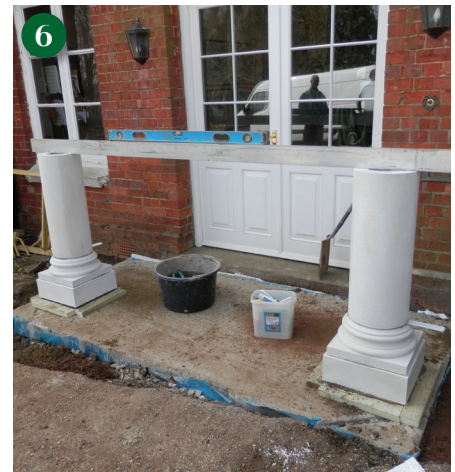
It is important to check levels throughout the installation process.
