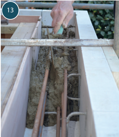
Concrete infill underway.
