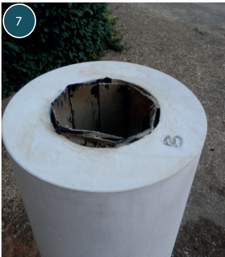
7 Polystyrene/Styrofoam (or similar) should be used to act as an isolating medium between the stone and infill concrete.
