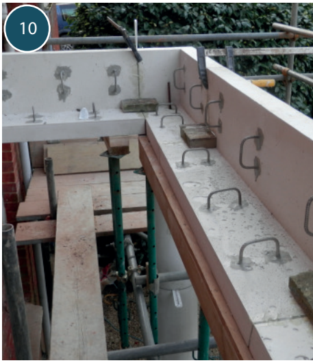
Entablature in position showing 'D' lugs.
