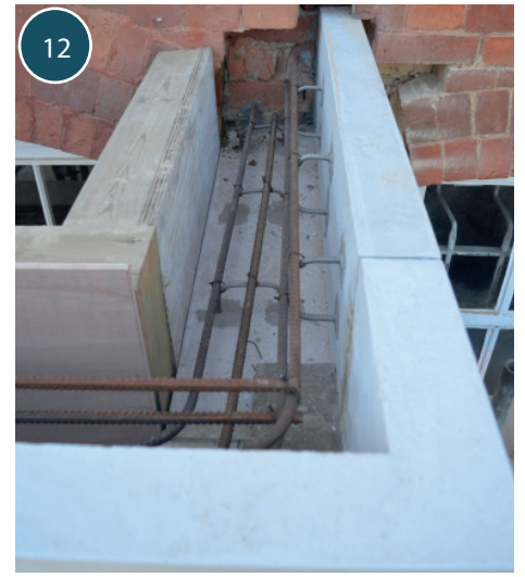
Entablature with steel reinforcement and shuttering in place before concrete infill (designed by others).
