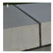
Before pointing ensure each 6mm  $(\frac{1}{4})$  joint is free from loose particles. Avoid pointing in extreme conditions, particularly wet and cold.
