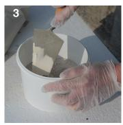
The cement and aggregate should first be mixed together dry in the ratio of 1 part cement to 4.5-6.5 parts aggregate.
