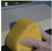
Wipe over the surface of the joint and surrounding area with a dampened sponge to remove all surplus pointing material off the surrounding areas and ensure a flush finish to the joint.
