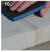
Any mix residue may be rubbed away with fine abrasive paper 2-3 days after completion.
