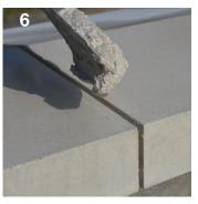
Scoop the mix into the joint, pressing with a trowel to ensure an even fill.
