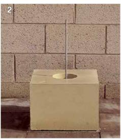
The column should be erected on a suitable The pedestal is then bedded on 1:1:6 cement/ The column base is bedded on the pedestal as Foundation, concrete and steel lime/sand mortar. All joints would normally be previously described. reinforcement to be designed by others to suit 6mm (1/4") with the mortar slightly recessed from loadings and ground conditions. Shown is a the surface of the stonework to allow for pointing
