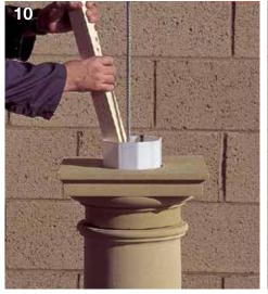
The isolating medium is then trimmed flush. Column ~ Entablature or Structure above: the Continue concrete infill until level with top of joint around the structural core between the capital. The capital is now ready for the next capital and the entablature or structure above stage, either (11) or (12).
