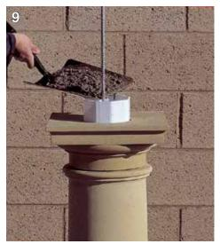
The capital is then bedded. The isolating medium is inserted into the core. The core is then partly infilled with concrete as previously described
