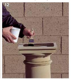
Column ~ Freestanding or timber pergola: the top of the capital will need to be waterproofed, as a minimum, with bituminous paint (applied in accordance with manufacturers instructions) to approximately 25mm (1") from the edge of the
