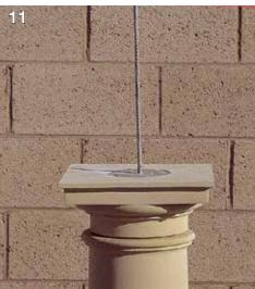
should be formed using a compressible filler, or a weak mortar mix, to form a 6mm (1/4") soft joint. This ensures that any loading is carried by the central structural core and not by the stonework.
