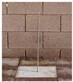
suitable steel starter bar set into a concrete after the column is erected. foundation.
