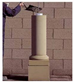
The bottom shaft section is then bedded and the isolating medium inserted as previously described. The concrete is again infilled.
