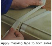
of the joint, keeping the tape approximately 1mm (1/16) from the edge of the joint.
