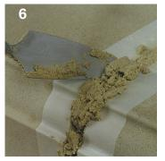
Scoop the mix into the joint, pressing with a trowel to ensure an even fill.
