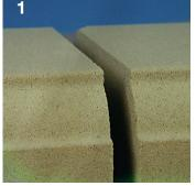
Before pointing ensure each 6mm (¼") joint is free from loose particles. Avoid pointing in extreme conditions, particularly wet and cold.
